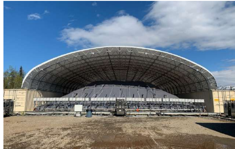
Ex-situ PFAS Thermal Conductive Heating (TCH) on 2,000 yd3 of PFAS impacted soil at Joint Base Elmendorf Richardson (JBER) in Alaska
