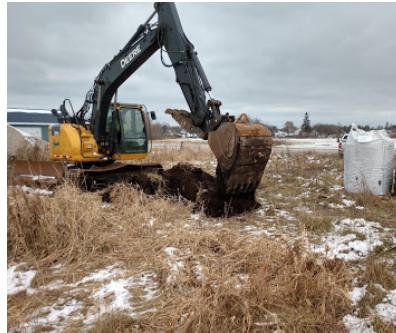
Excavator based soil mixing
